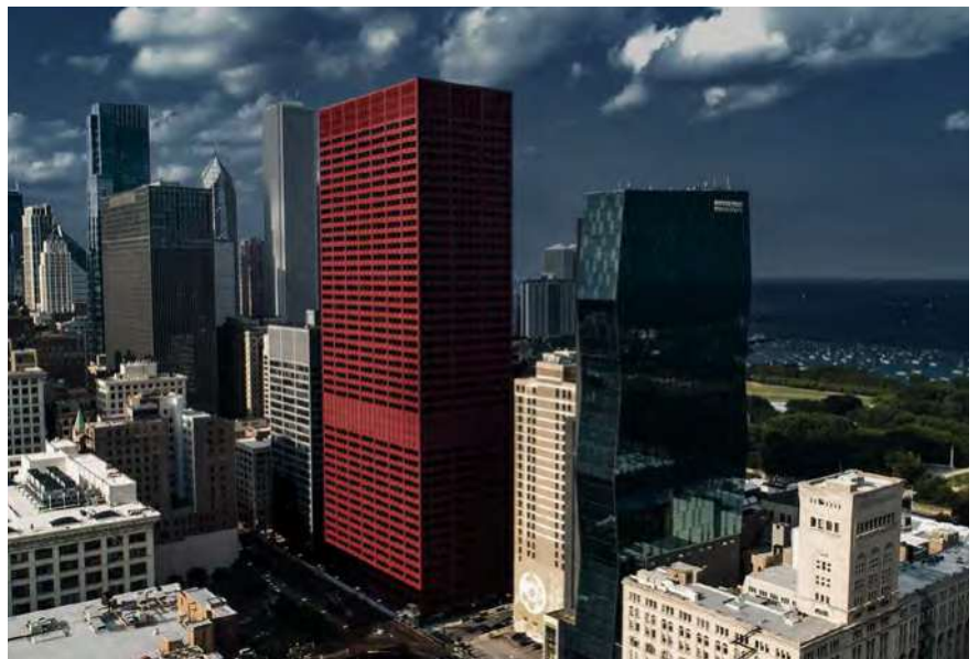
„BIG RED“ PRIME OFFICE TOWER – CHICAGO
